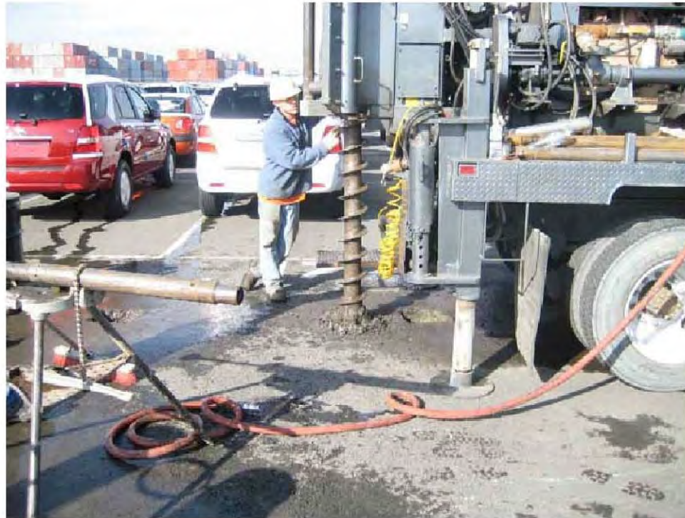
Photo 1. Drilling boring SC-1.
